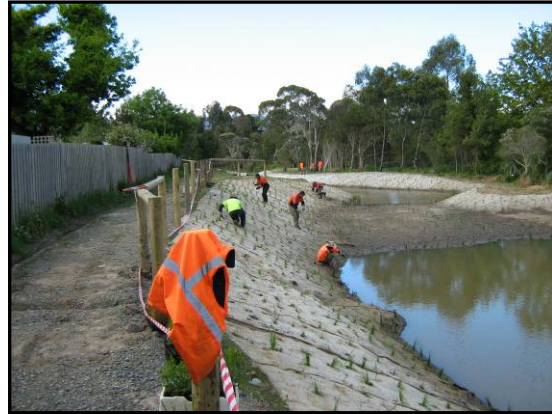
Revegetation planting along the newly built flood protection channel during Stage One
